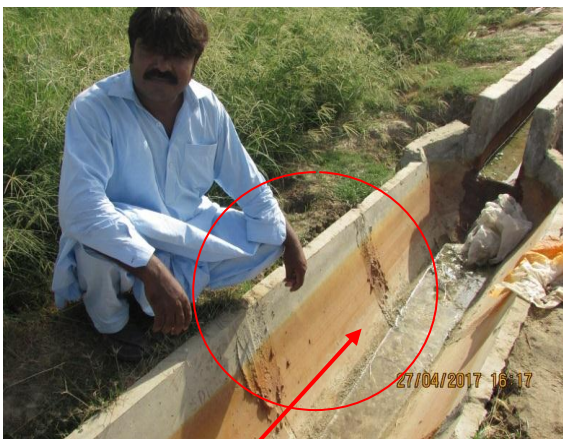
Substandard Plaster
