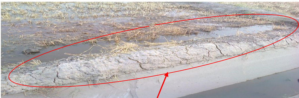
Mud support to compensate decreased depth of watercourse
