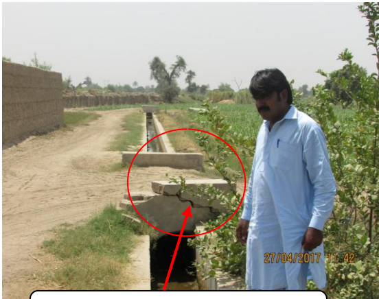
Broken culvert
