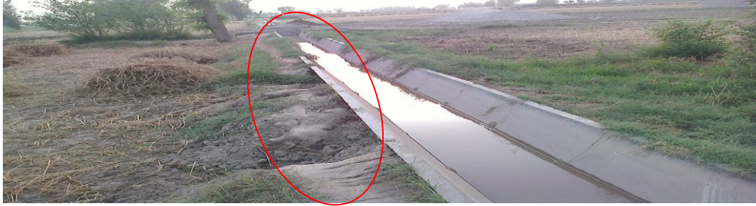
Watercourse No. 128/13/4 Machka Tehsil Sadiqabad
